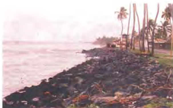
Coast protection measures to protect coastal erosion - Hendala Wattala- West Coast
